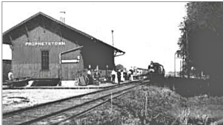
Our 1871 railroad depot.
